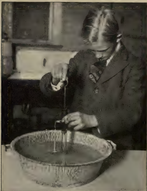
FIG. 9. A glass model suction pump.
